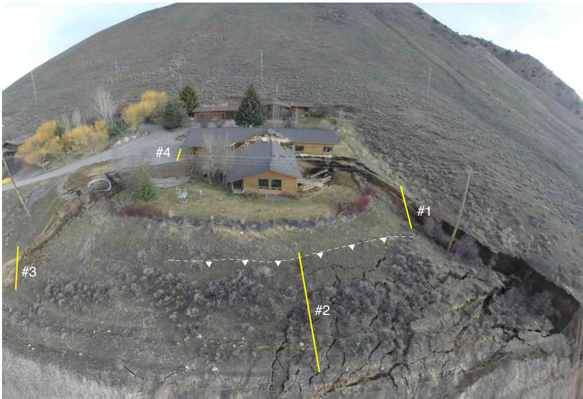
Figure 3 Arrangement of extensometers across head scarp fissures. East Gros Ventre Butte, Jackson. The northern slump block which has severed the house has thrust beneath the fissured central graben block immediately to its south monitored by instrument #2 (green trace in Figure 4).
